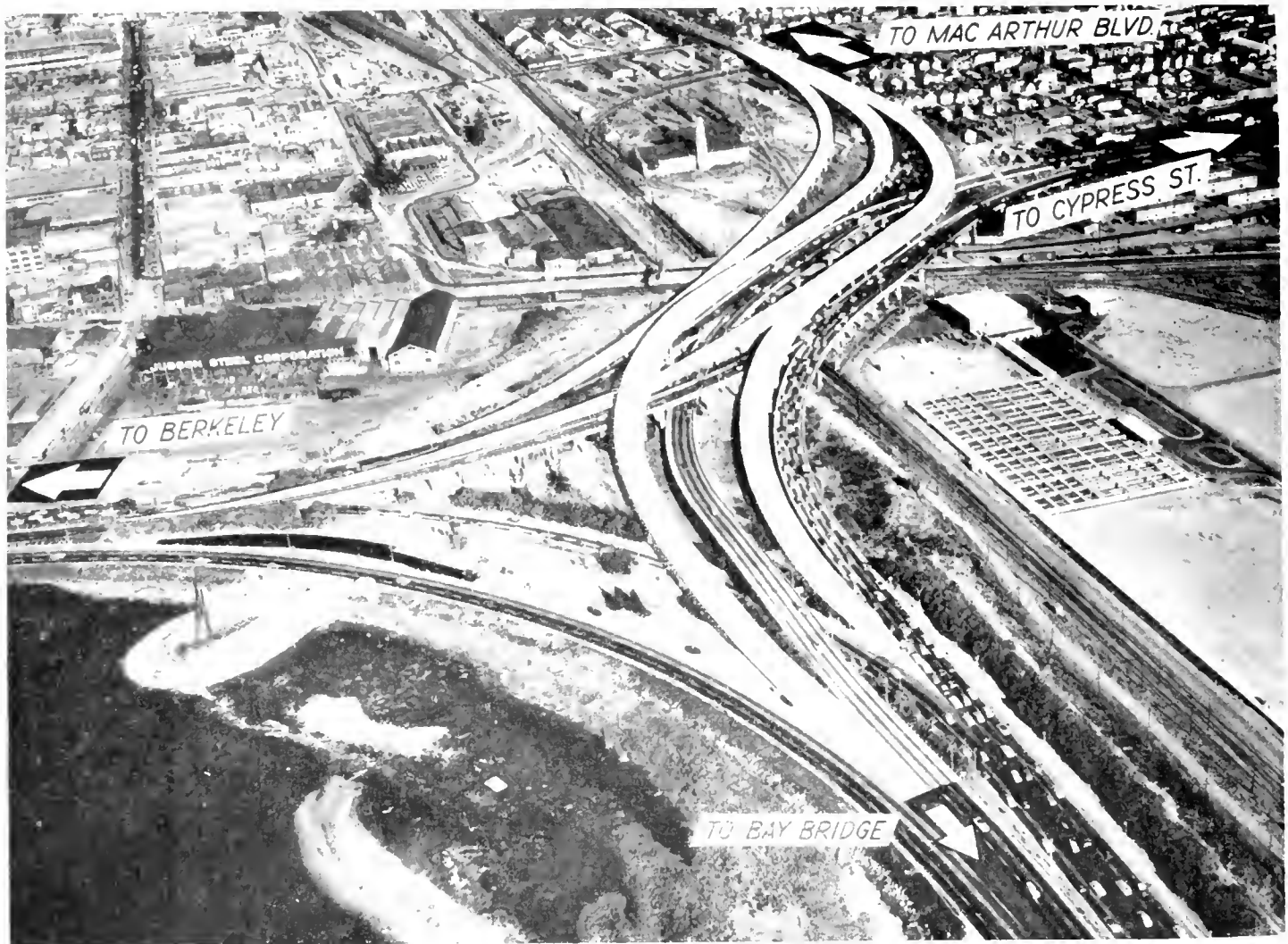
Engineers drawing of improved East Bay traffic distribution structure in Oakland. A third-level ramp is being built over existing traffic lanes connecting the San Francisco-Oakland Bay Bridge with MacArthur Boulevard. A curved ramp will be added from MacArthur Boulevard to the Eastshore Freeway. The improvements will double traffic capacity and are designed to eliminate cross-weaving traffic.
